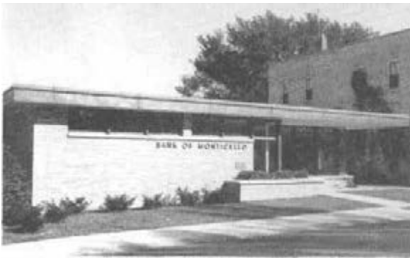
The bank of Monticello is located in this building constructed in 1959.
