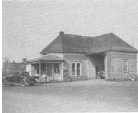
The original lumber yard office.
