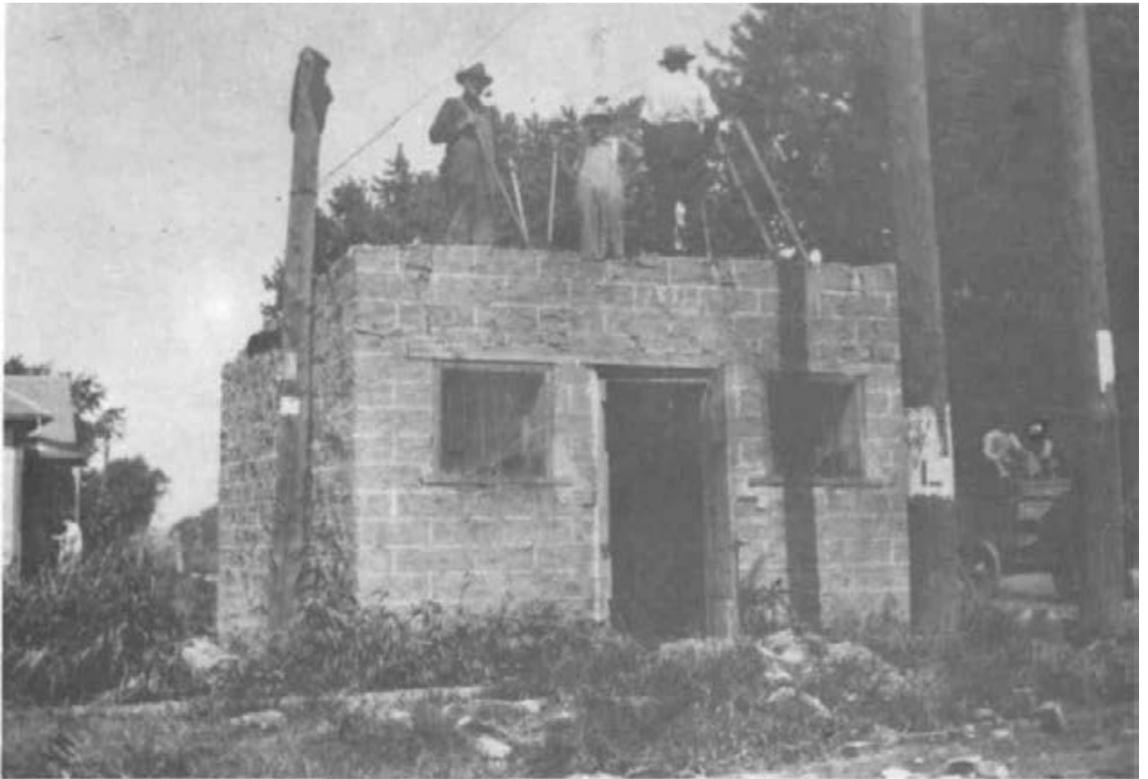
The old jail as it was being torn down.
