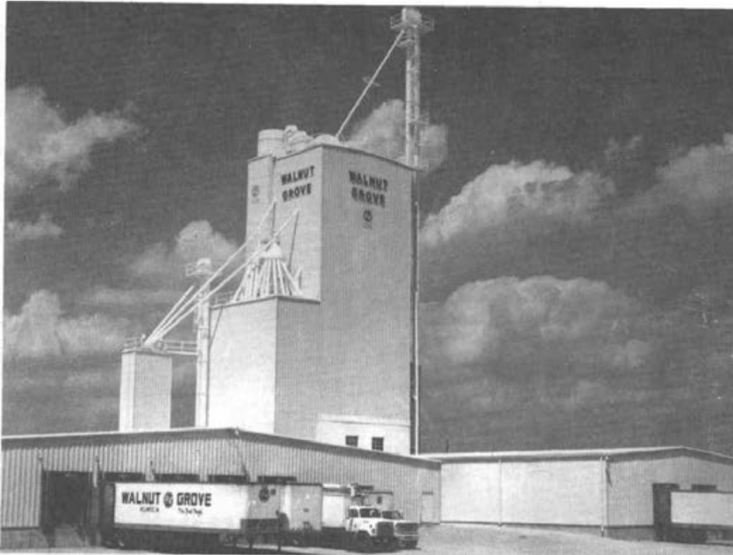
The Walnut Grove (4x4) plant in Monticello.
